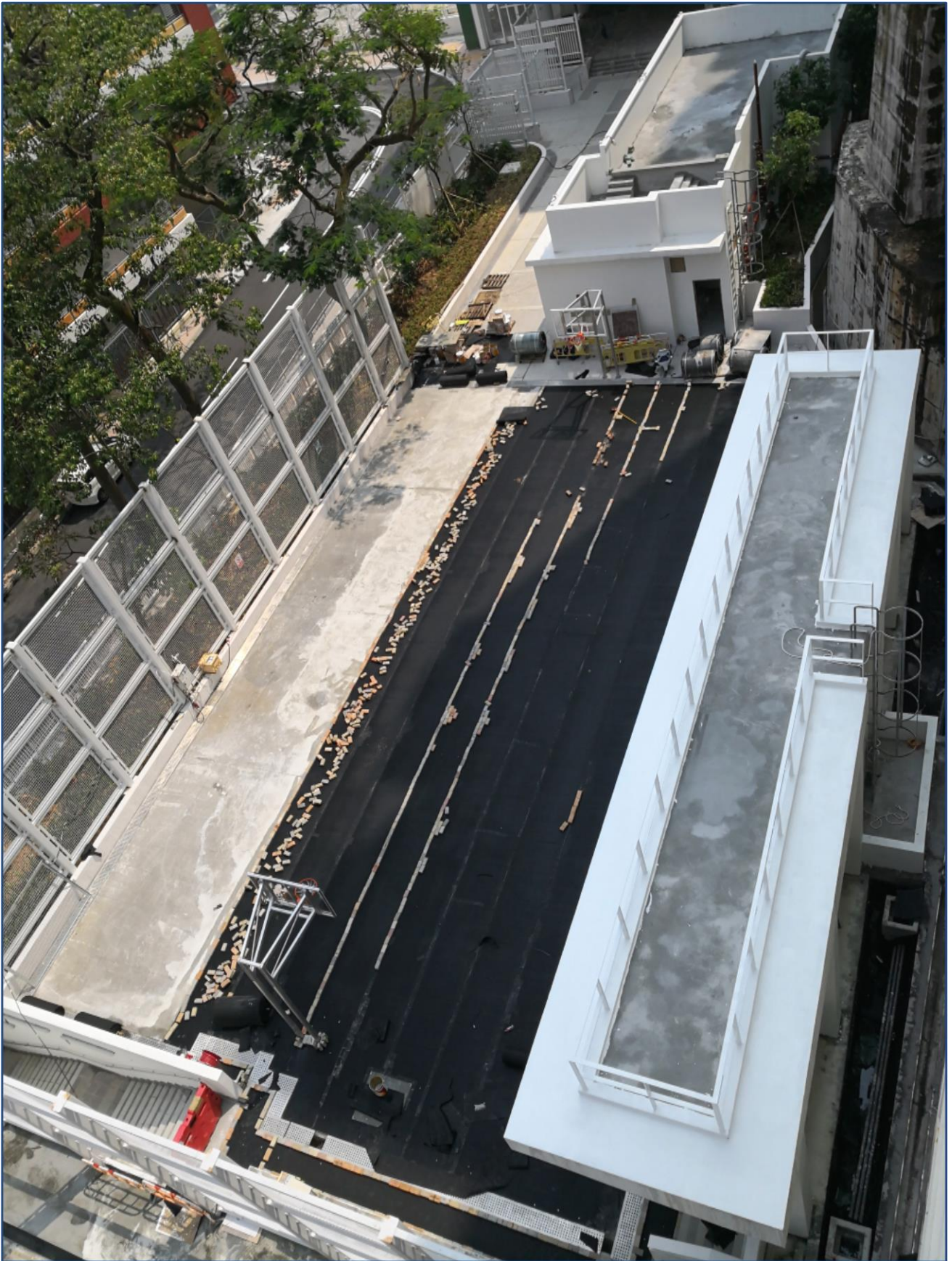
Laying mattress at ball court in progress
