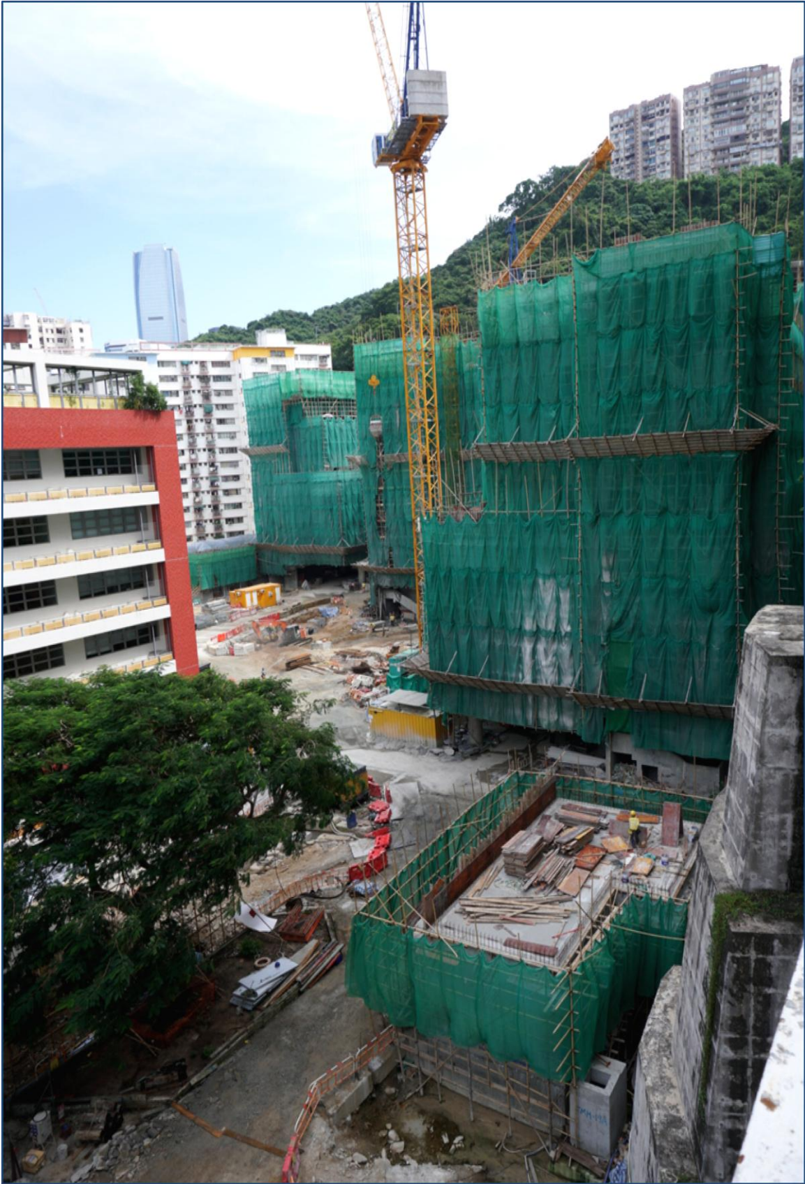
HV Room, Transformer Room and LV Room – Construction in progress
