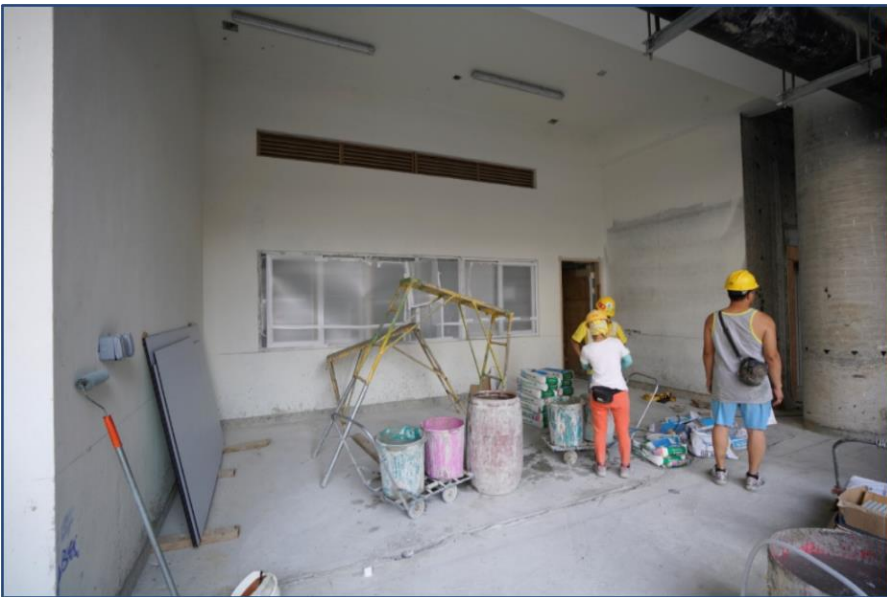
Area in front of Guidance Activity Room
