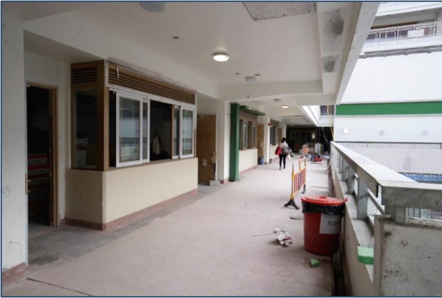
2/F Classrooms at East Wing
