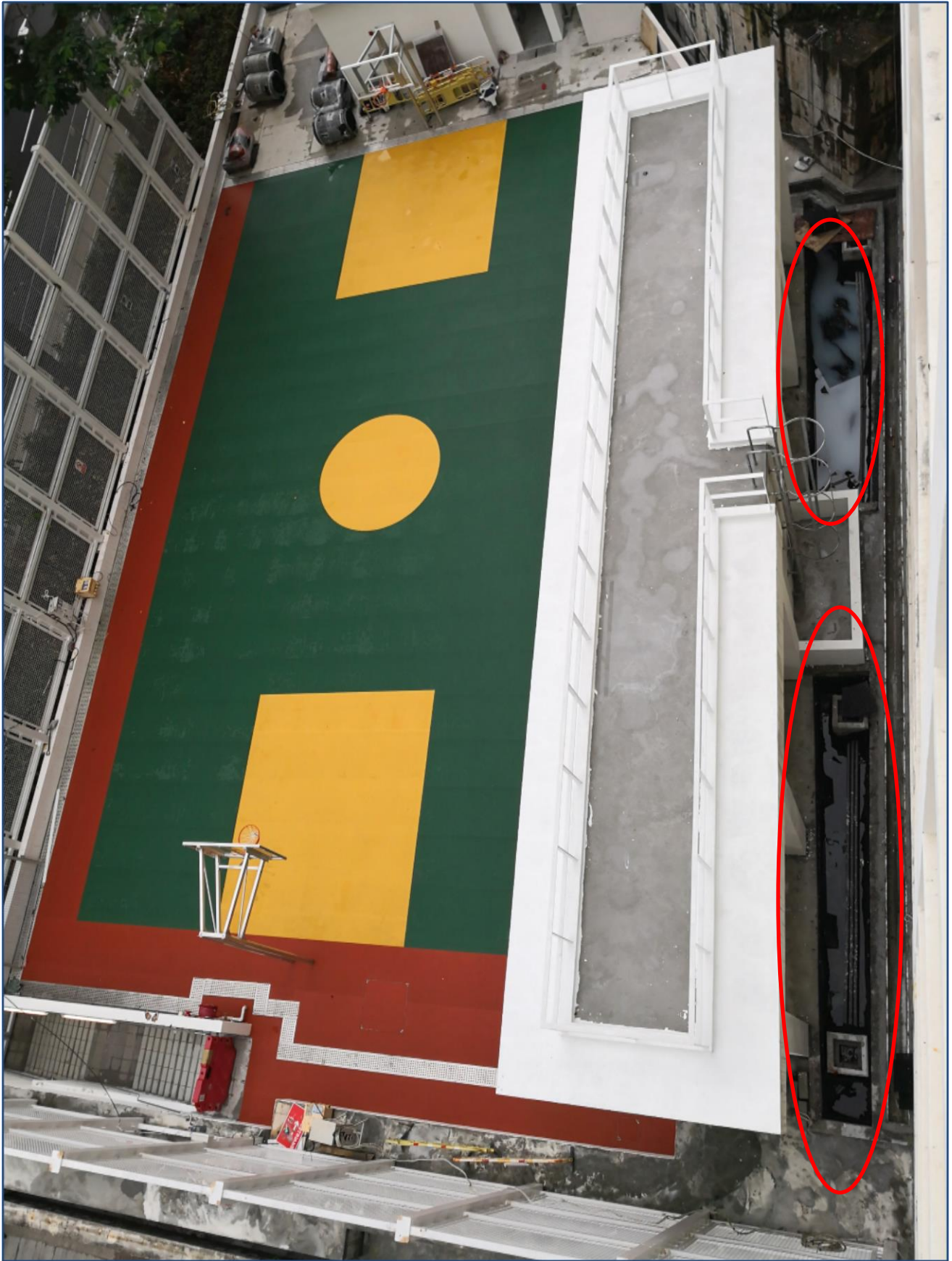
Laying mattress at ball court completed
