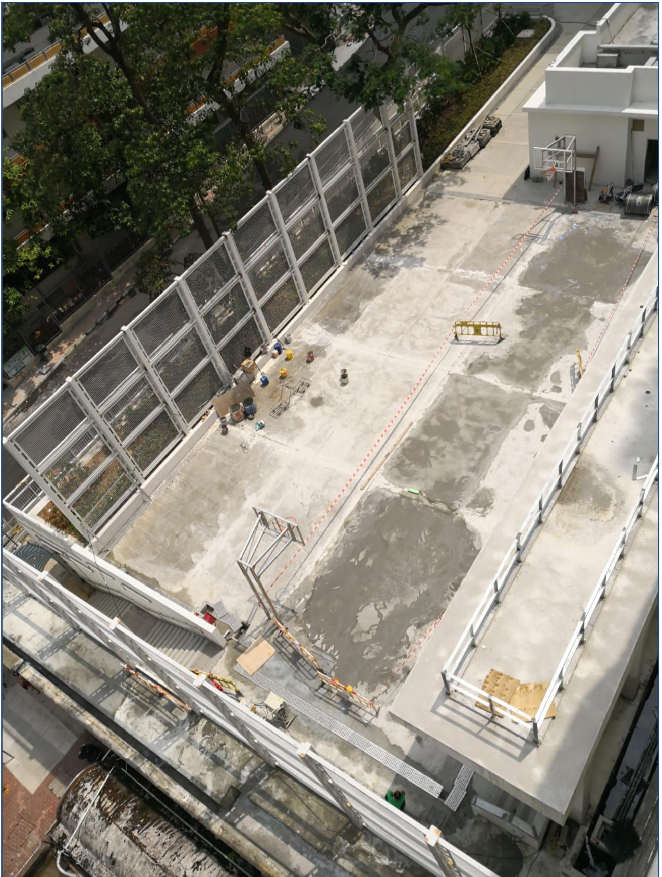
Ball Court – Preparation for laying mattress
